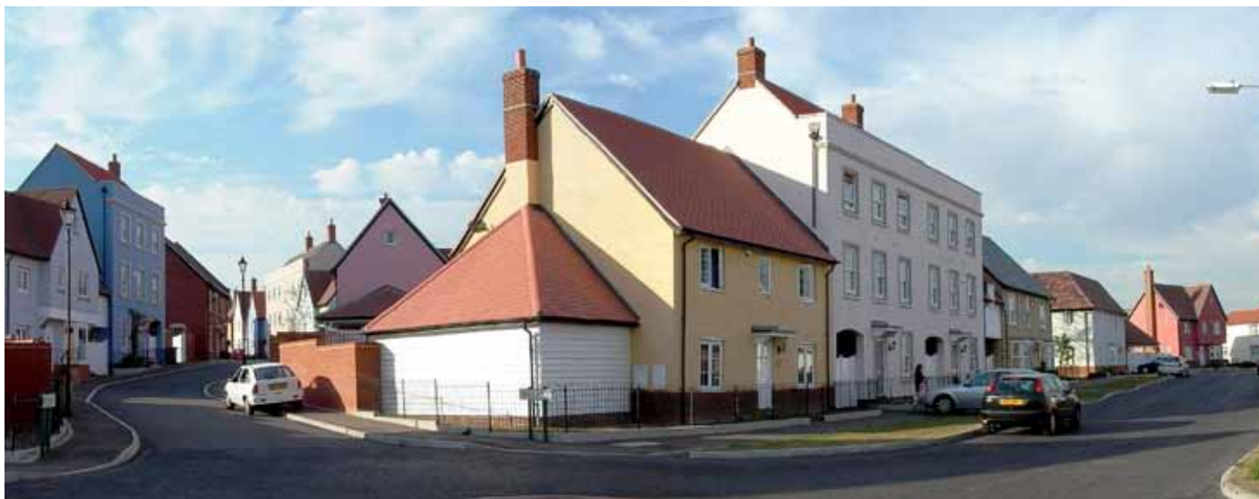
42. Networks should be direct and visually open, with the main public routes for all users fronted and overlooked by homes.
