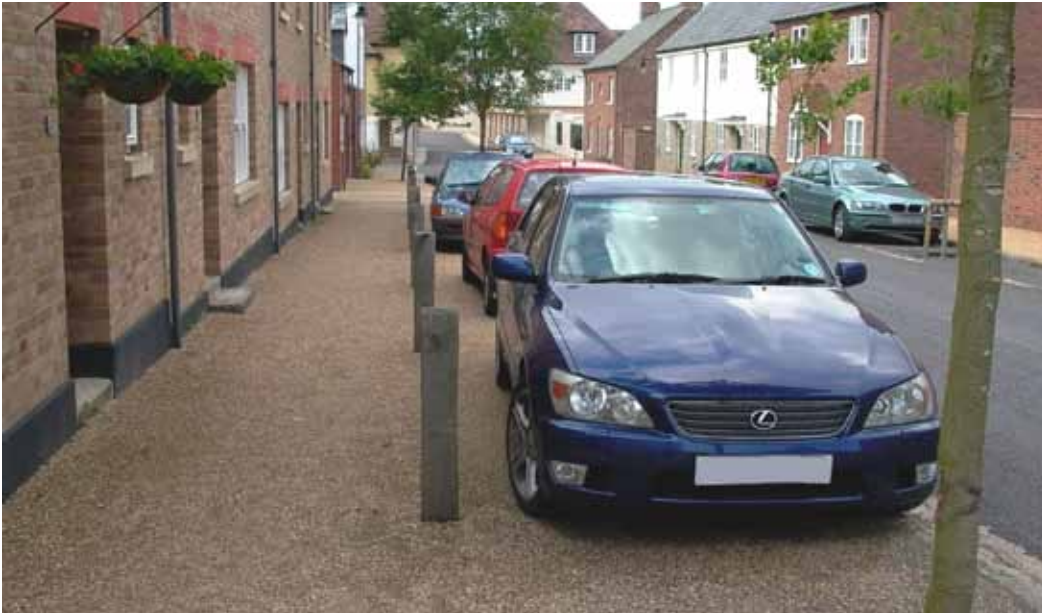
60. Visitor parking should be located close to homes, and on or close to the street.
